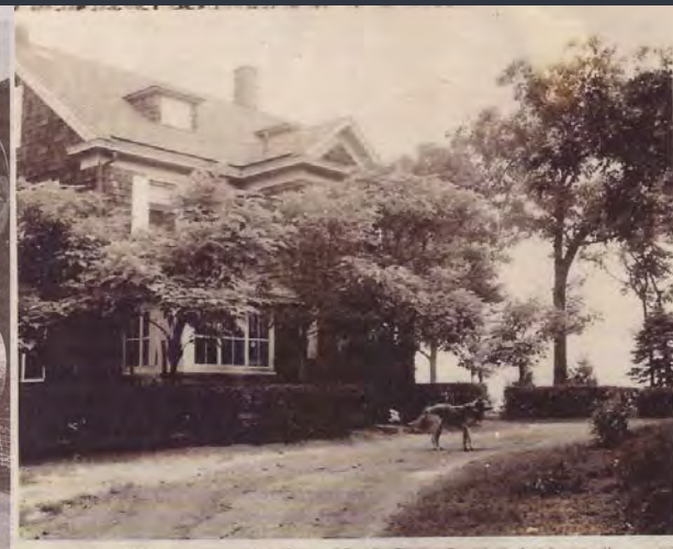
THE HOUSE PROPER IN WHICH THE UNDERCOVER STATION IS LOCATED. NOTE ABSENCE OF OUTWARD EVIDENCE OF RADIO ANTENNAS, FEED LINES, TOWERS, ET CETERA.
